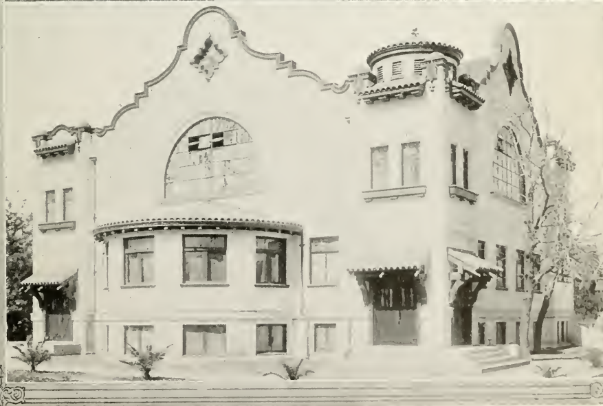
THESE BUILDINGS, A BANK, COUNTRY SCHOOL AND CHURCH, ARE REPRESENTATIVE OF THE PUBLIC AND BUSINESS PROPERTIES OF THE COUNTY
