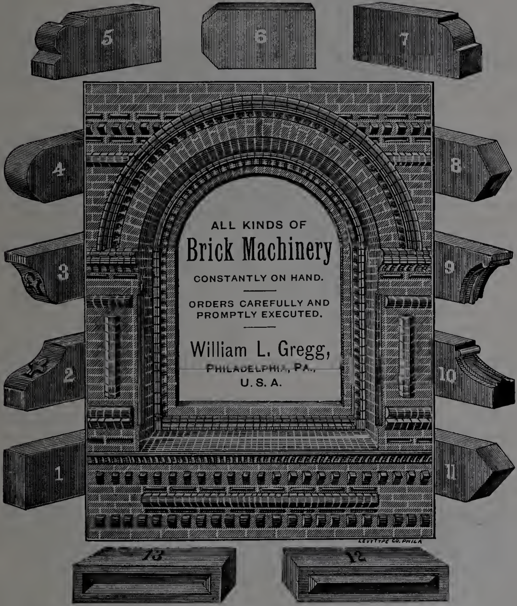
Ornamental and Front Brick made on the Gregg Machines.
