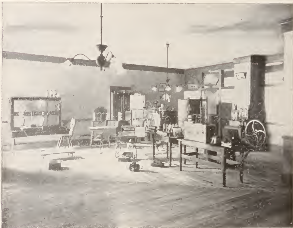
The electric current which supplies the building, passes from the electrolier, through a bank of lamps on a table in the center of the room, to the various electrical devices.
