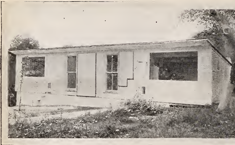
Curtain-front Poultry House used by J. W. Parks, Altoona, Pa.
