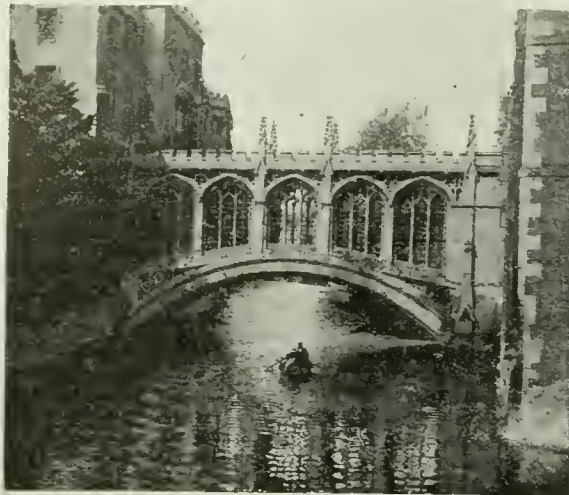
THE "BRIDGE OF SIGHS," ST. JOHN'S COLLEGE.
