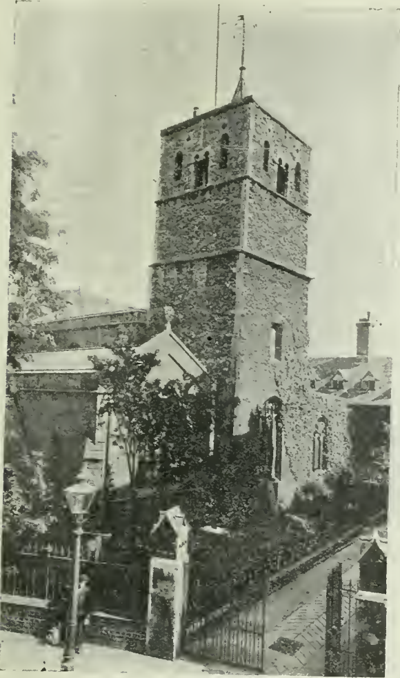
SAXON TOWER, ST. BENET'S CHURCH.
