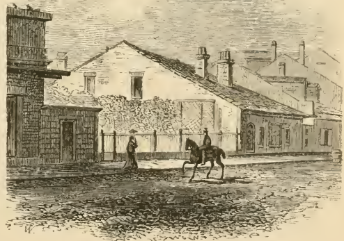
"Some aged private dwellings, rapidly decaying."
