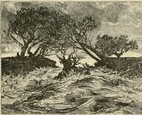
A Crevasse in the Mississippi River's Banks.
