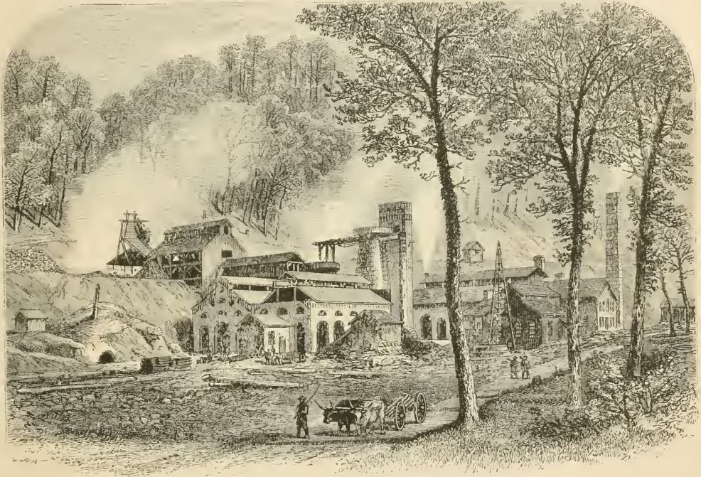
The Rockwood Iron-Furnaces—Eastern Tennessee.
