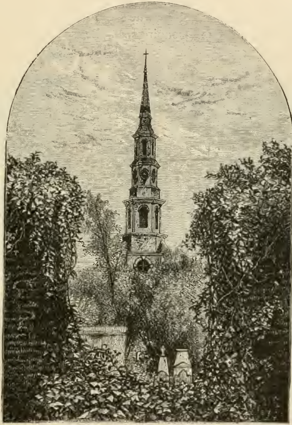
The Spire of St. Philip's Church—Charleston.
