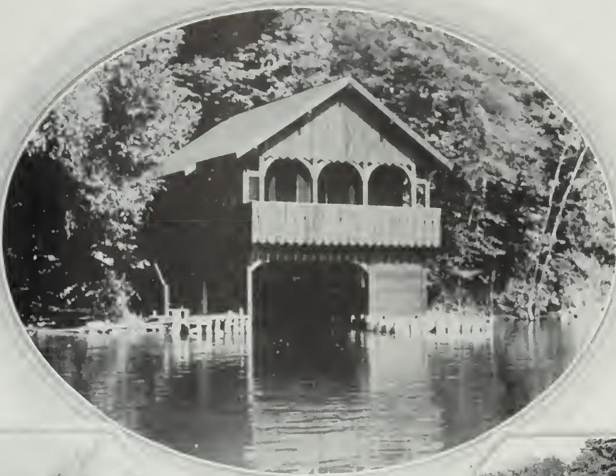
The Wickwire boathouse at Lake Skaneateles is attractively simple in construction, and amply large to meet the summer boating needs of the average country place on the water
