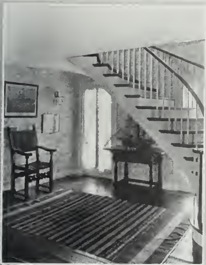
Above. The hall, showing the elliptical free-standing stair, behind which French doors provide access to the paved court
