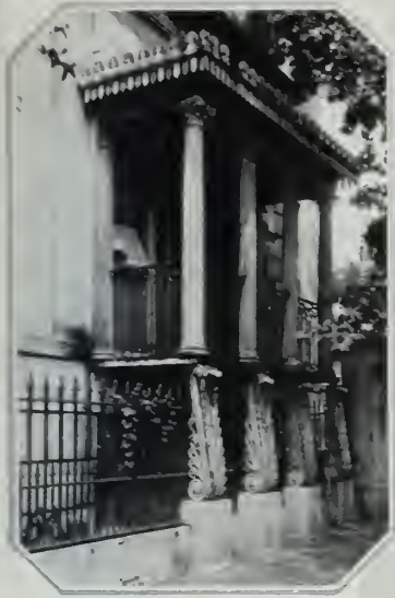
Above. This entire balcony, including pedestal consoles, columns, etc., is of cast iron, indicating the wide range of the use of this material in the nineteenth century. House in Savannah, Ga., about 1830
