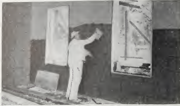
A preparation of cork insulation in board form to which the plaster may be directly applied
