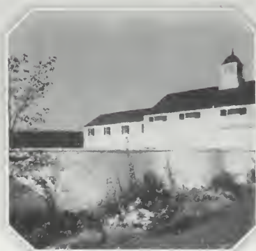
manner in which the short ridge of the original farmhouse roof was lengthened by placing the chimney outside the walls is clearly shown. At left, a glimpse of the barn over the hollyhock-bordered wall
