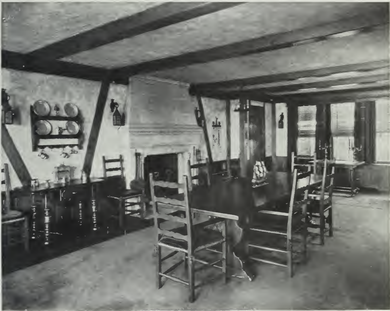
DINING ROOM of rough oak and modeled antique plaster. Mantel of Verdun stone. Furniture of both Oak and Walnut specially designed
