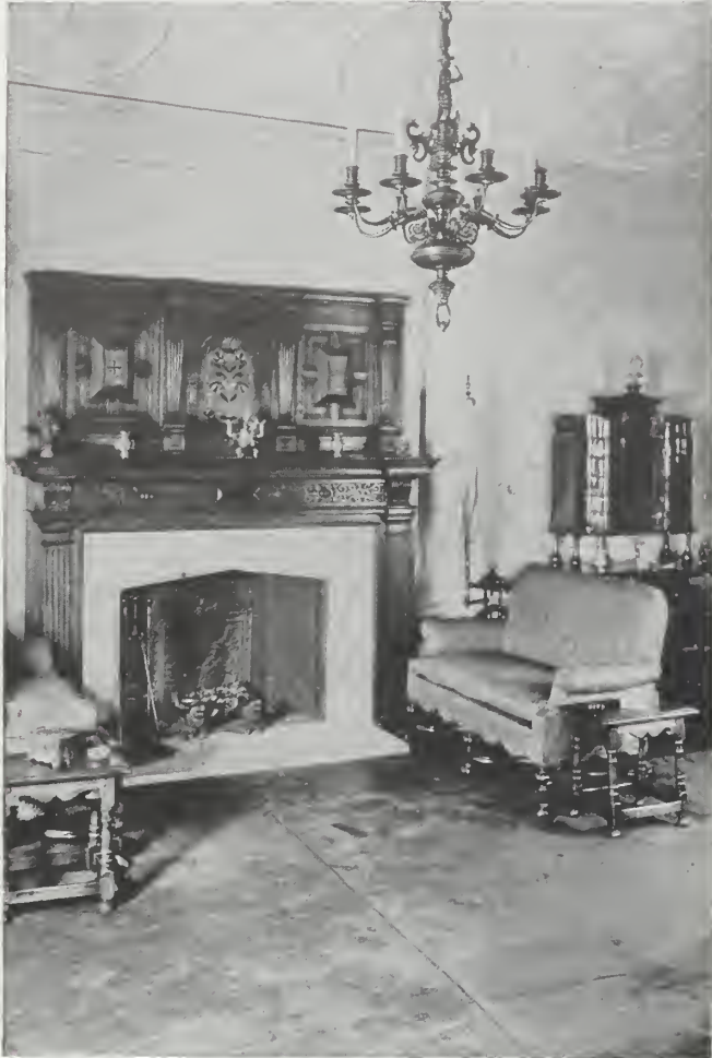
Living Room with Mantel of Carved and Inlaid Oak and Stone Facing and Hearth. Interior Designed and Carried Out Completely by
