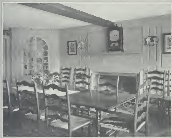
The dining room in the original stone house, showing the summer beam partly revealed through the plaster, indicating its origin during the transition from the period when a summer beam was completely exposed (as in the living room) to the later custom of entirely concealing it behind plaster
