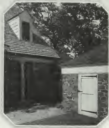
Left. The stonework which flanks the service porch harmonizes with the original masonry of the old smoke house, the door, cornice, and roof of the latter being restored
