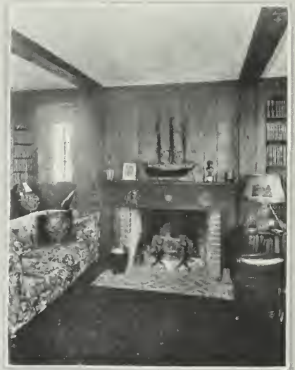
In the pine-walled study the mantel, posts, and ceiling summers are hand-hewn chestnut from an old barn on the place
