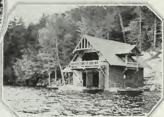
Dormer balconies insure airiness to the second floor of this attractive boathouse at Burnt Rock Camp
