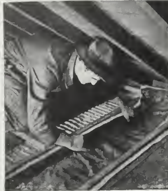
A flexible wool-like preparation from wood, with paper covering, that can be tucked snugly into corners and around windows
