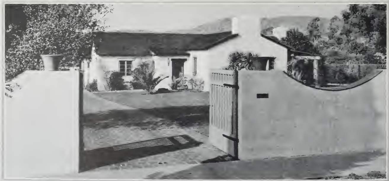
The outside walls are white stucco, and the exterior trim is stained a weathered gray, matching the color of the roof of hand-split shakes. Dark red tile roof-ridges and hips and green-painted window sash complete a delightful exterior color scheme
