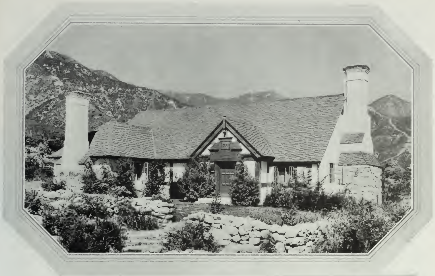
In the Falconer residence an effect entirely different from that attained in the Behr bungalow is achieved by the steeply pitched roof. The chimney treatment is especially attractive, featuring a combination of natural stone and painted brick
