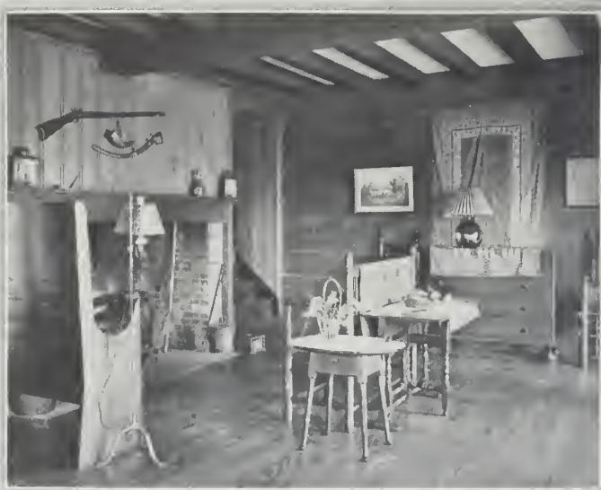
Detail of the living room. The huge fireplace was reproduced from a contemporary example in the Metropolitan Museum of Art, with its old vertical pine boards and antiquated molding. Note the horizontal pine sheathing on the farther wall, and the wide oak plank floor.
