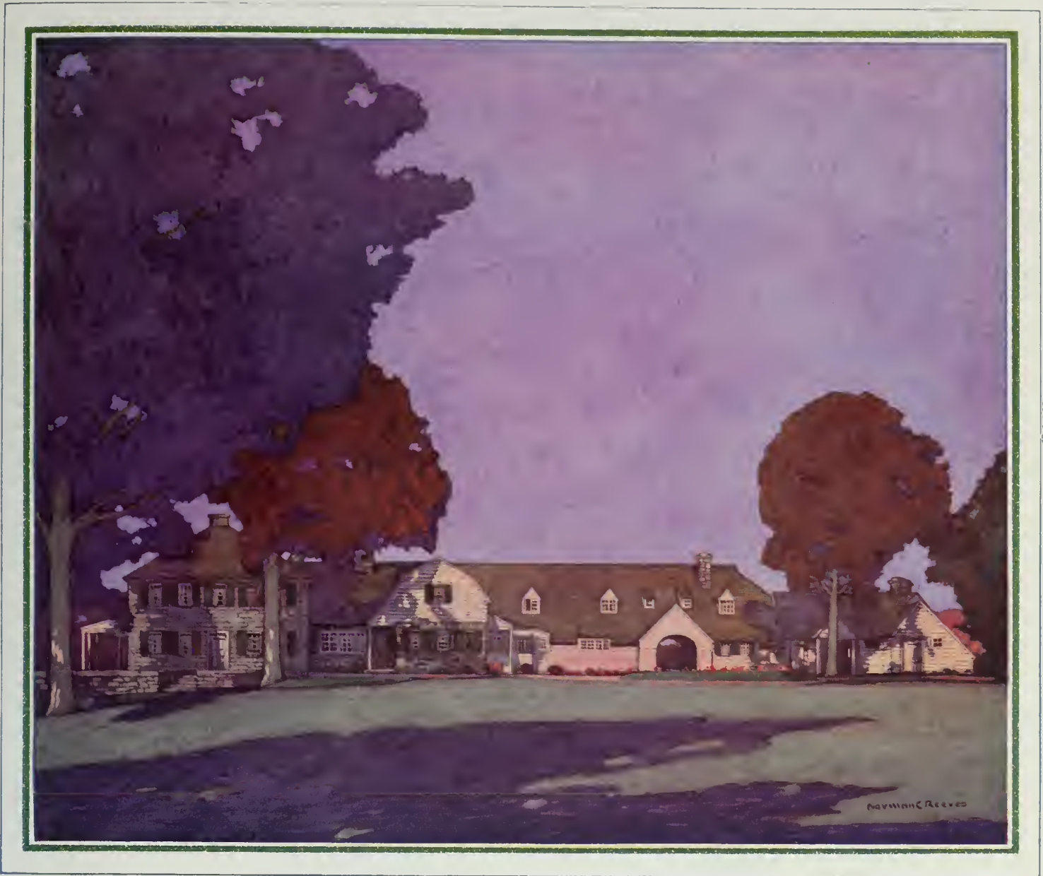
The front elevation, showing at the left the original stone building with its hip roof. The gambler-roof unit is part of the new work carried out in the old manner
