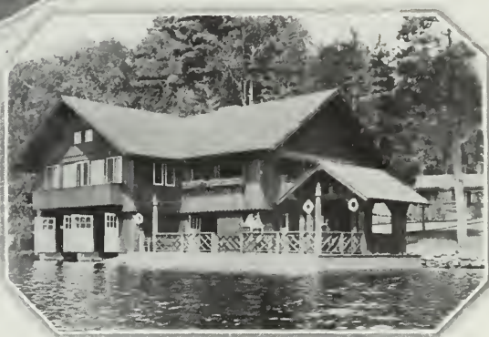
The same boathouse shown at left, as it appears from the water side
