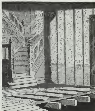
Mineral wool used as insulation for floor and walls. Note in the wall the installation of wire lath over the insulating material
