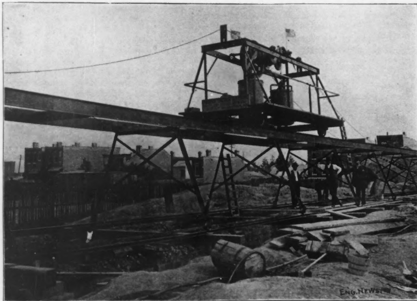
VIEW OF THE POTTER TRENCH MACHINE. Potter Mfg. Co., Indianapolis, Ind., Makers.
