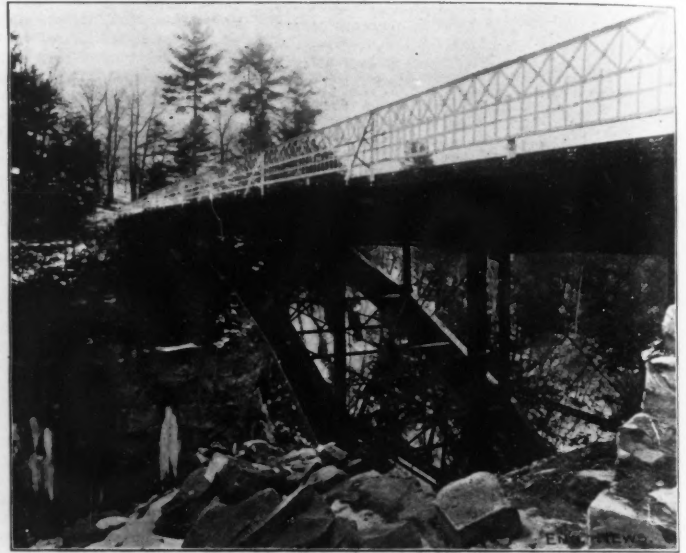
Fig. 2.—End View Showing Arch Ribs and Bracing.
