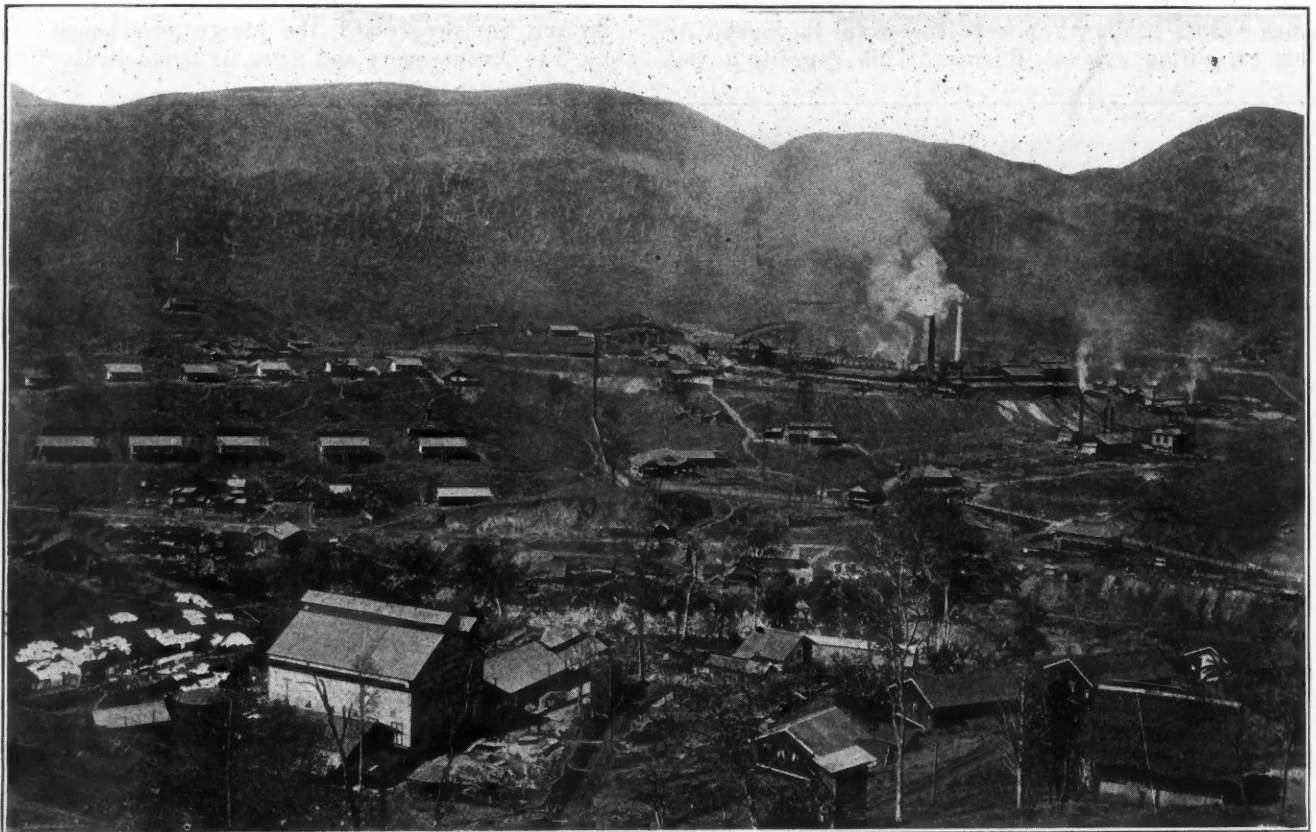
LEAD SMELTER AND REFINERY, LOOKING SOUTHWEST
