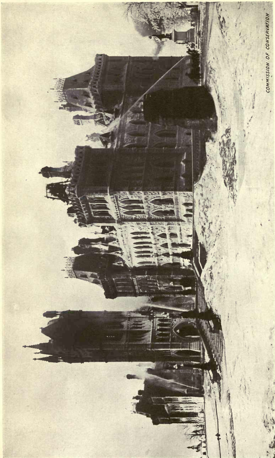
DESTRUCTION OF CANADA'S PARLIAMENT BUILDINGS, OTTAWA, FEB. 3, 1916 Fire-resisting walls often hide highly combustible interior construction.
