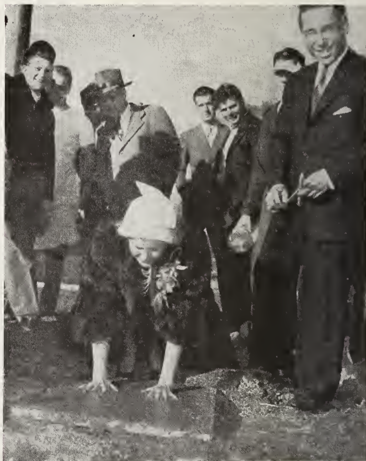
DEDICATION of the forthcoming prefabricated Crest theatre, St. Louis. Virginia Mayo, actress, impresses her handprints into concrete which will be a sidewalk block at the theatre's entrance. Norman Probst, owner, is at the right. The house will have television and a milk bar.
