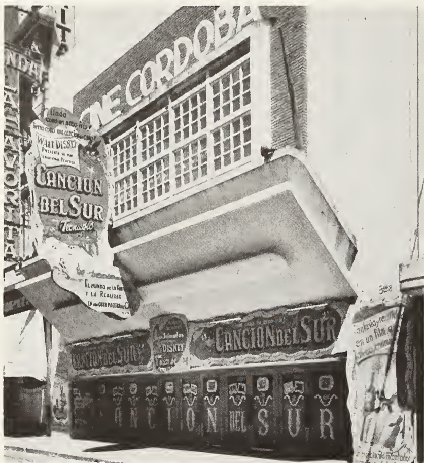
The Cordoba theatre in the Argentine key city of San Rosario displays front for Walt Disney's "Song of the South". Note the angle of the marquee which contains concealed indirect units to flood exterior with no visible source of light (above).
