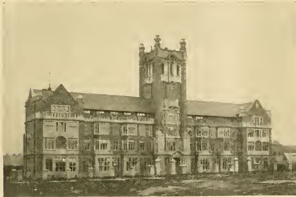
FIG. 1.—New front wing (facing west) of Armstrong College, to be opened by the King on July 11. In the centre is the Sir Lowthian Bell tower.
