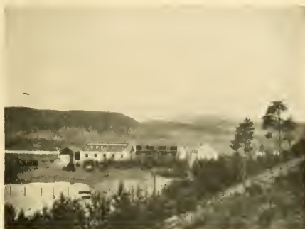
FIG. 1.—View of nitric acid factory at Notodden.
