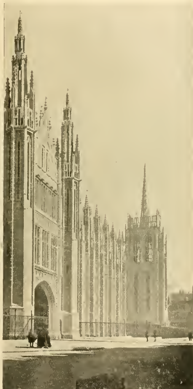
FIG. 2.—Front of Marischal College Buildings, looking southward.
