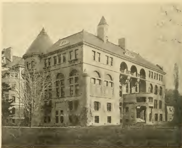
FIG. 1.—Macdonald Physics Building, McGill University, Montreal.
