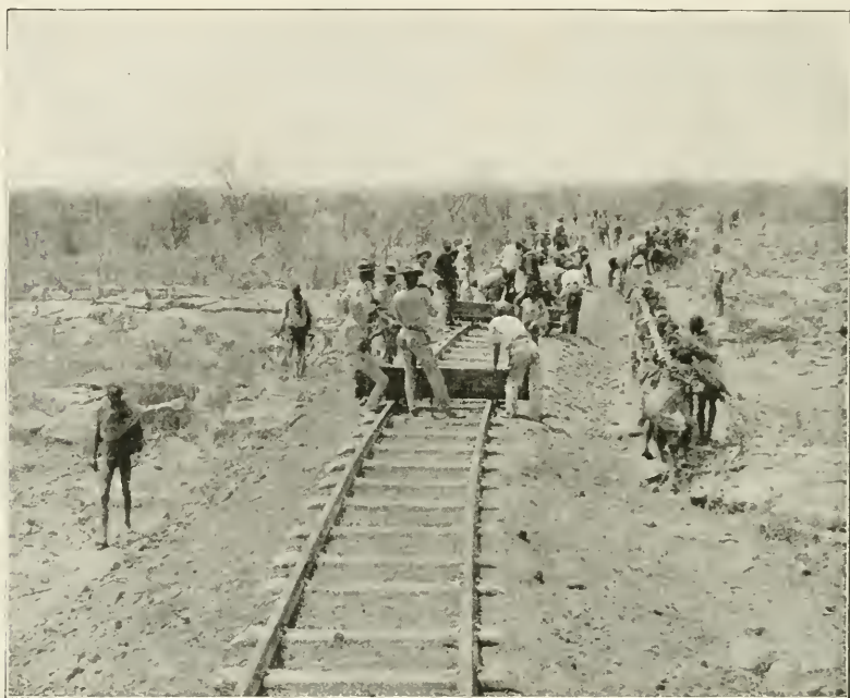
CAPE TO CAIRO RAILWAY. LAYING THE RAILS
