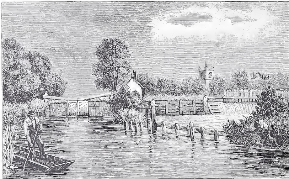
No. 11.—Benson Lock and Weir.
