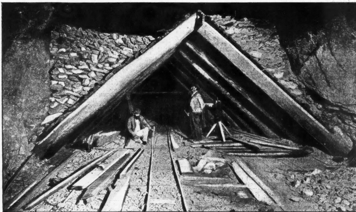
TIMBERING IN KALGOORLIE MINE, WESTERN AUSTRALIA.
