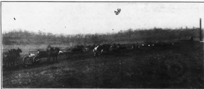
REMOVING OVERBURDEN, PHOSPHATE MINE
