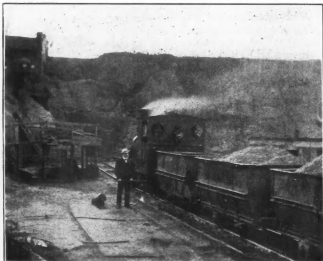
FIG. 2. SHOWS DUMP CARS HAULING FILLING MATERIAL FROM DREDGE TO MINE
