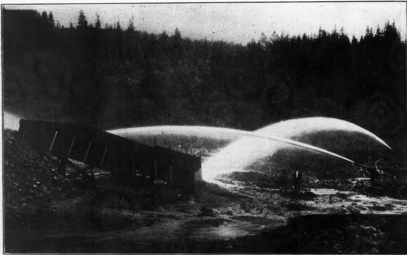
RUBLE GRAVEL ELEVATOR. ONE GIANT HANDLING BOULDERS, ANOTHER SUPPLYING MATERIAL
