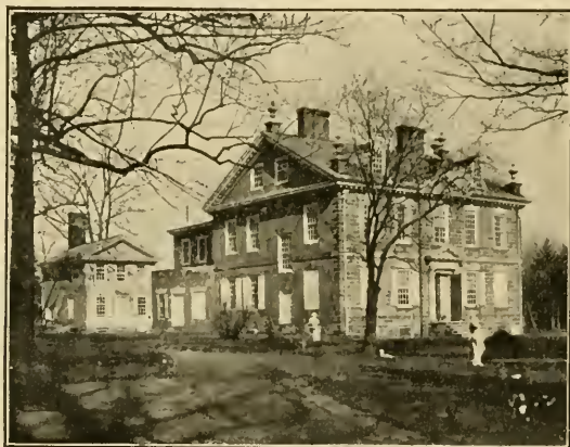
A COLONIAL HOUSE AT GERMANTOWN, PENNSYLVANIA.
