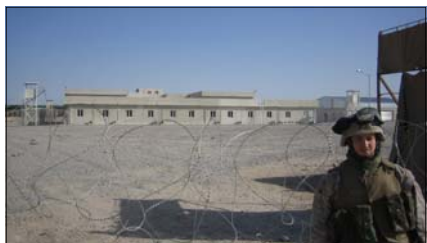
Cpl Thrift standing in front of completed Iraqi Police Station.
