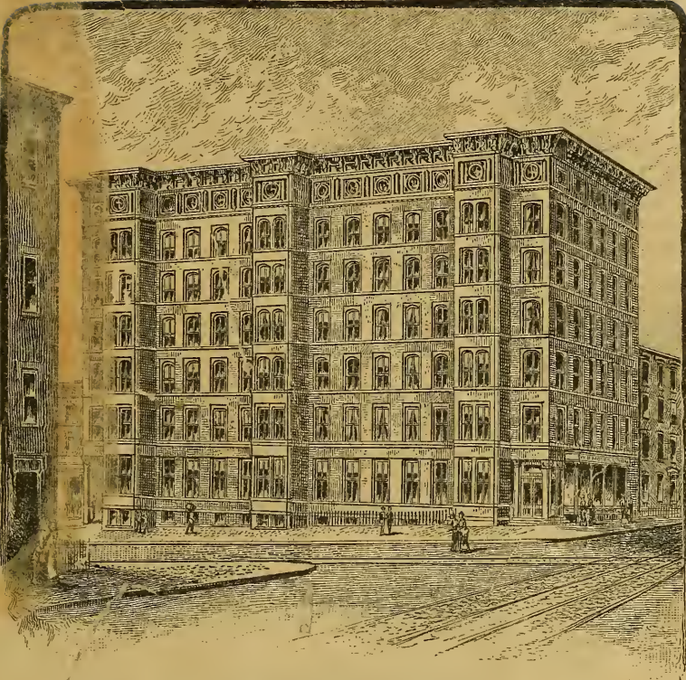
THE W. B. MOSES BUILDING.
