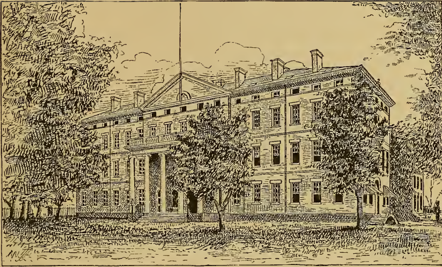
OLD WAR DEPARTMENT BUILDING.
