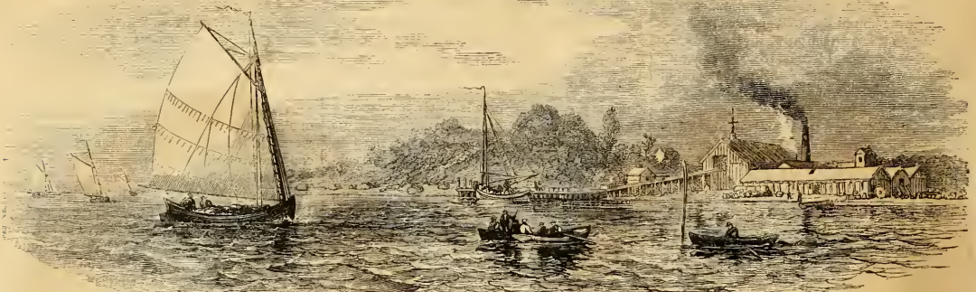
Fig. 1.—VIEW OF THE FACTORY WITH A LOADED "CARRYAWAY" RETURNING.
