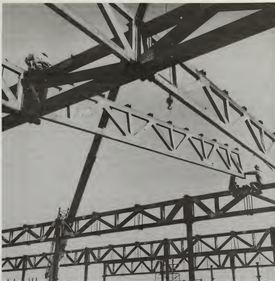
Engineered wood structural members are used frequently in nonresidential structures. (Credit: USDA Forest Products Laboratory)
