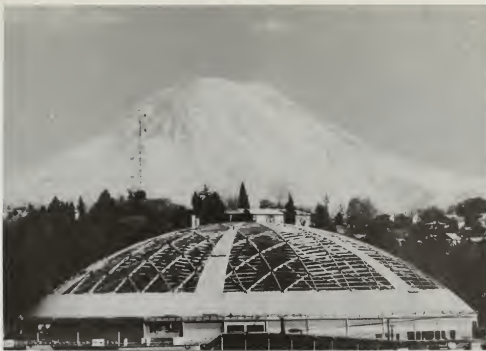
Wood is being increasingly used in large nonresidential structures such as the Tacoma Dome.
