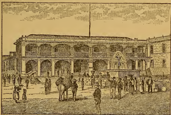
The Government Building, Quezaltenango.
