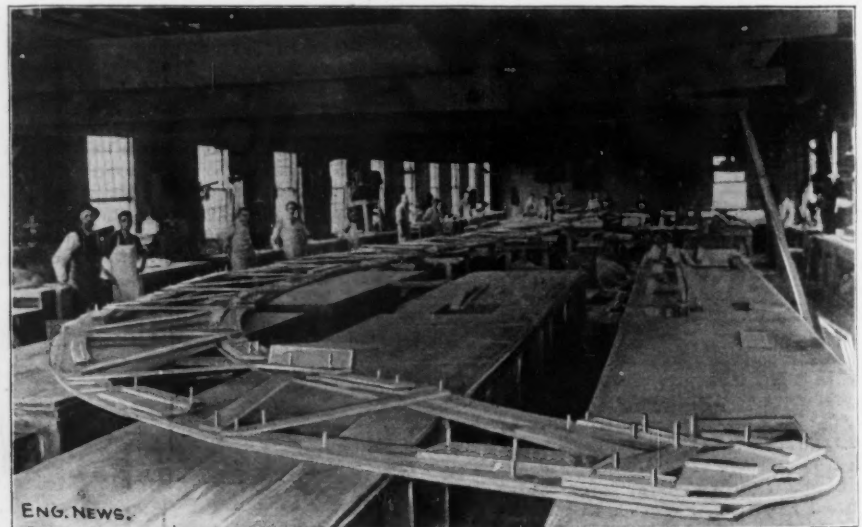
FIG. 3.—INTERIOR VIEW OF TEMPLATE SHOP AT ELMIRA BRIDGE WORKS, SHOWING METHOD OF LAYING OUT TRUSSES ON BENCHES; ELMIRA BRIDGE CO.
