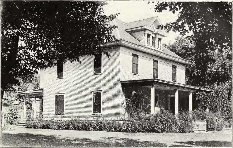
A York home showing the pleasing effect of proper banking of shrubs near the foundation.
