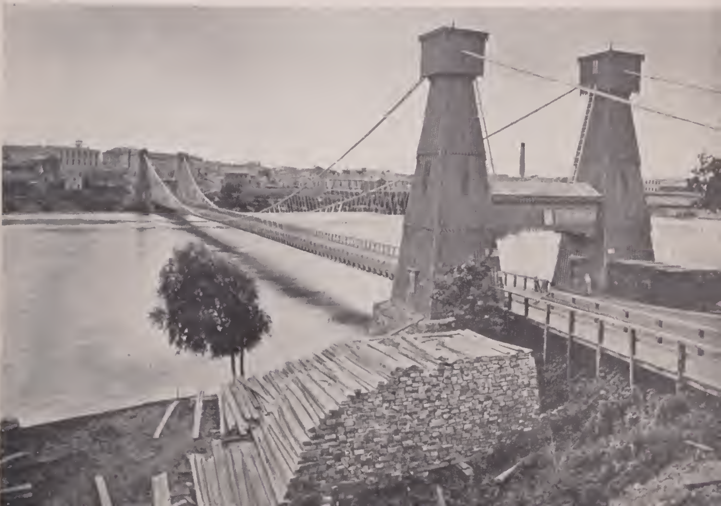
FIRST SUSPENSION BRIDGE
