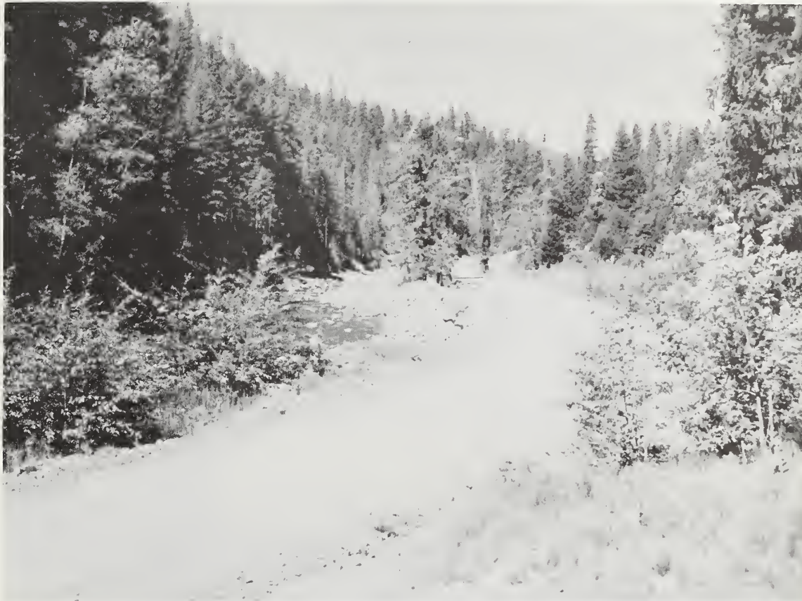
This road was constructed across an oxbow and is encroaching upon the stream.
