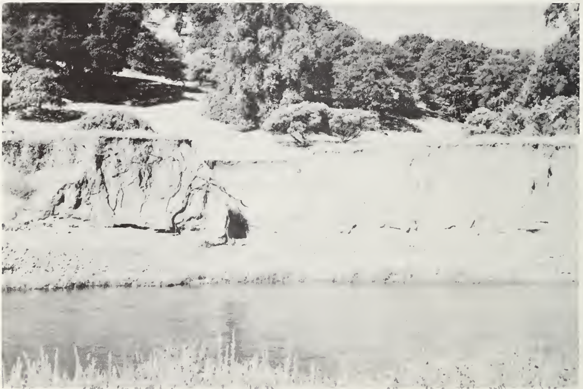
Streambank erosion along the Russian River. SCS PHOTO 3-5258-6
