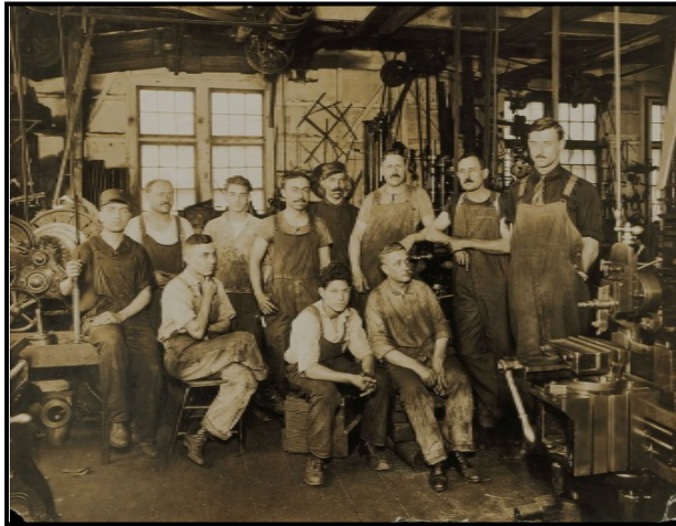
I. DeFrancisci & Son crew from 1917 in Brooklyn. This crew originally built the mixer, gramola and press. Pictured here standing right to left: Joseph DeFrancisci (tall man - Ignazio's son), Ignazio DeFrancisci & Cosimo Alati. Joseph Bontempi - sitting with hand under chin. Notice the overhead pulley system on ceiling with belt connecting to machine on left.
