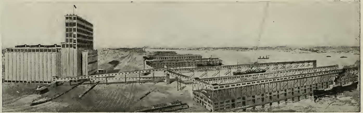
The Most Efficient Grain Handling Plant in the World
