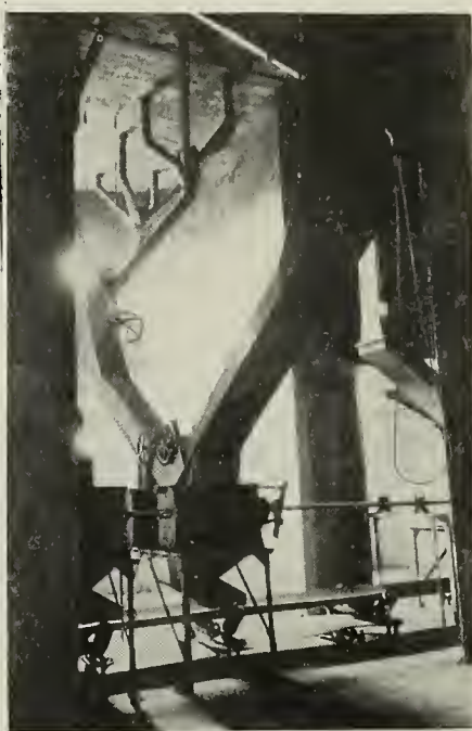
SPOUTS FROM FEEDERS IN NEW ELEVATORS
