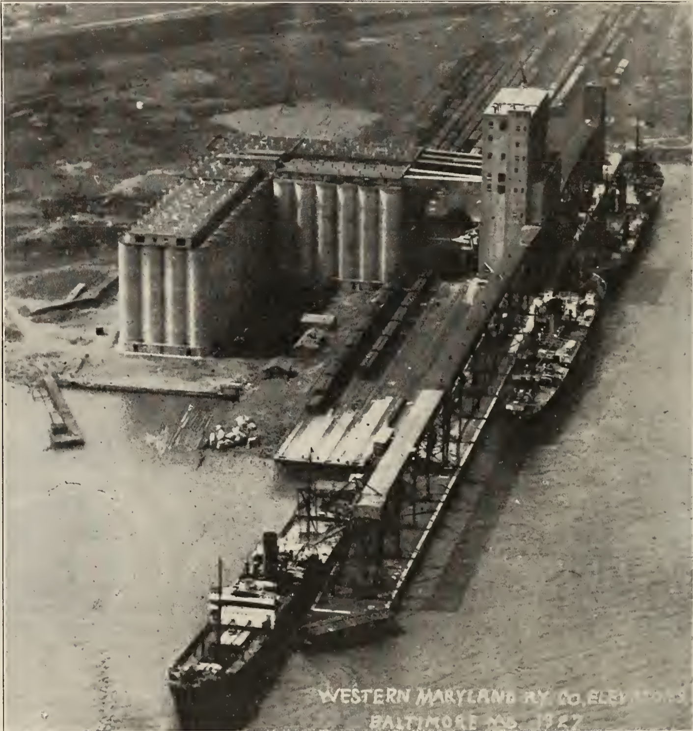
PORT COVINGTON ELEVATORS, WESTERN MARYLAND RAILWAY COMPANY, BALTIMORE, MD. CAPACITY 4,000,000 BUSHELS—EQUIPPED UP TO THE MINUTE
