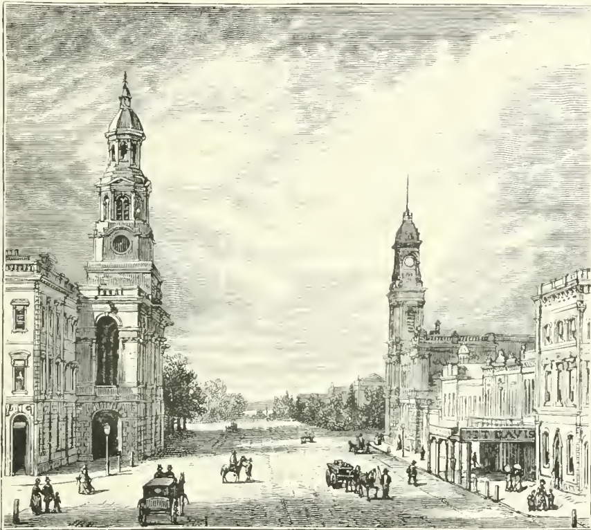
POST-OFFICE AND TOWN HALL, ADELAIDE.
