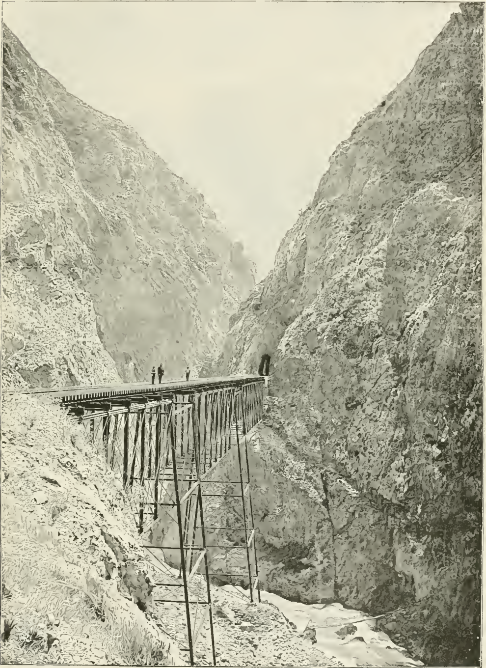
Fig. 7.—ANDES SCENEFY. VIEW TAKEN AT THE CHAUPICHACA BRIDGE, LIMA—LA OROYA RAILWAY
