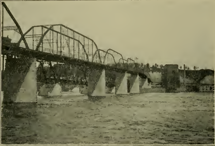
East Dubuque and Railroad Bridge.
