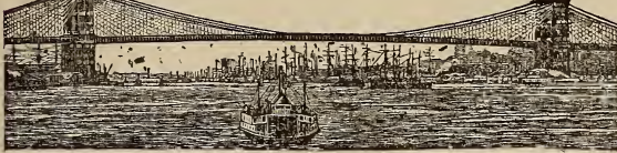
New York and Brooklyn Suspension Bridge: total length, 5,989 ft.; river span, 1,695.6 ft.; completed in 1883.
