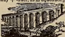
Viaduct of Masonry.
