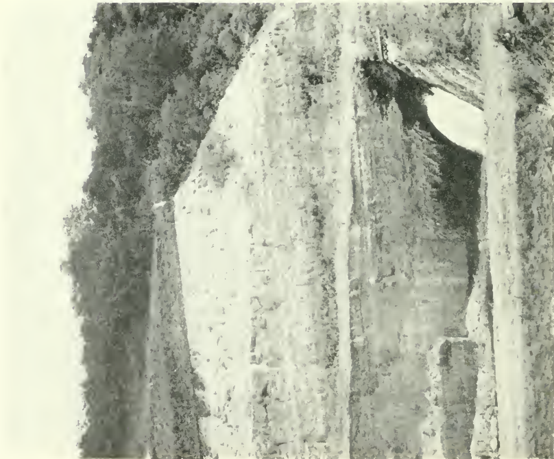
Varying geology along the Canal is emphasized by formations in the Third Locks Cuts. Left, Gatun sandstone at Atlantic end; right, columnar basalt at Pacific end.
