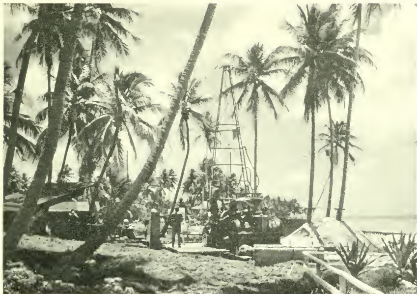
1. THE G. E. FAILING CO. DRILLING A DEEP HOLE ON BIKINI ISLAND, 1947
