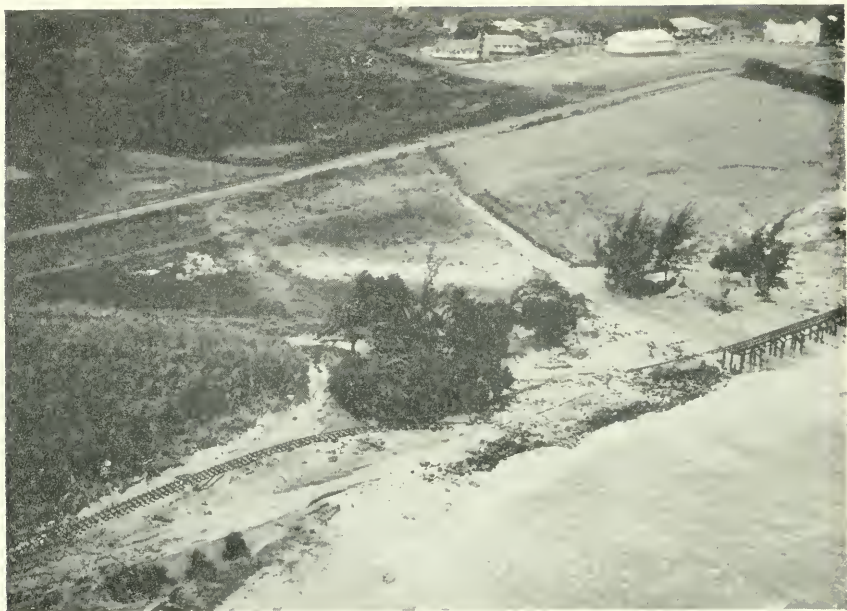
1. RAILROAD TRACK SWEEPED INLAND FROM ITS BED AT WAIALEE, OAHU Photograph by U. S. Navy.
