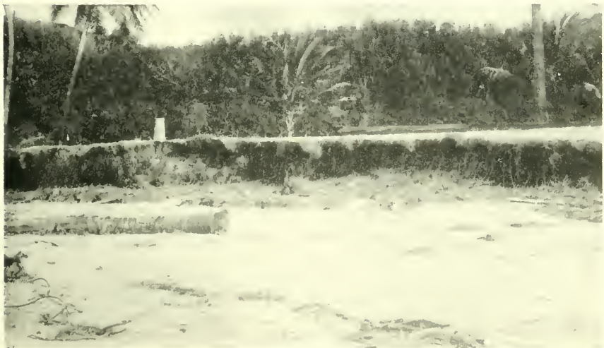
2. SCARP 5 FEET HIGH CUT BY THE TSUNAMI AT THE HEAD OF THE BEACH AT MOLOAA, KAUAI
