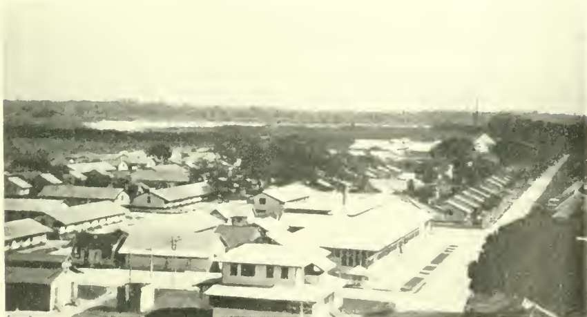
2. Moengo, Surinam. Practically every square foot of surface of these buildings was sprayed with a 2.5-percent wettable DDT powder.
