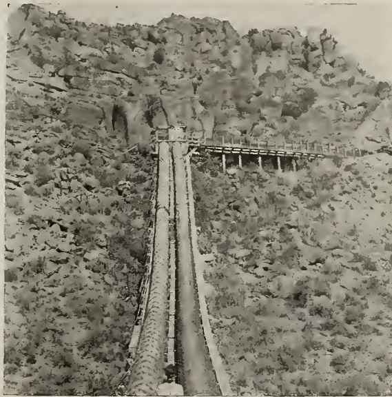
BIG SIPHON Irrigation System Cowychee Gap, Yakima Valley, Washington
