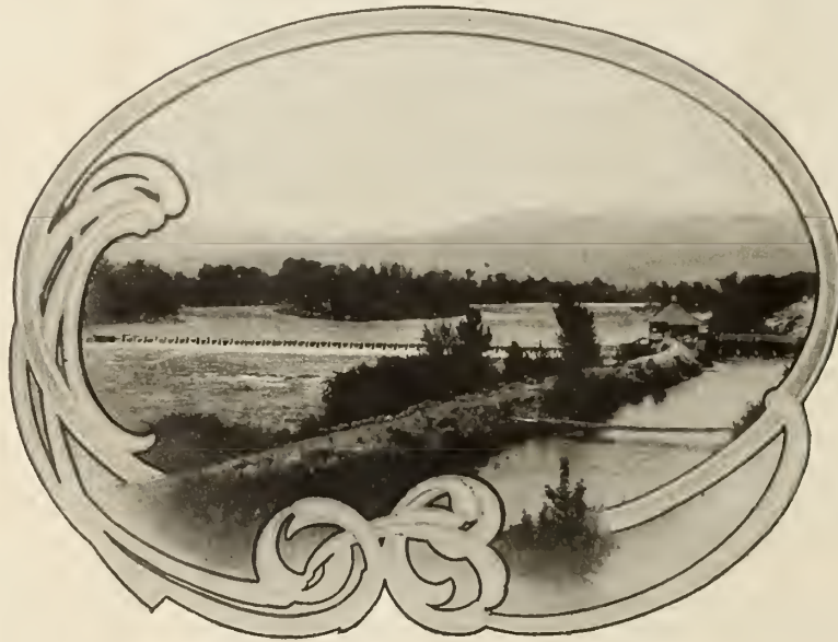
SUNNYSIDE CANAL HEADGATE, YAKIMA VALLEY
