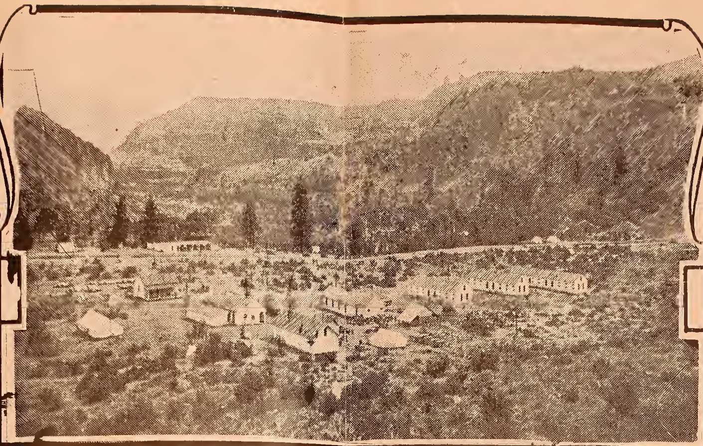
VIEW OF CAMP NO. 1, TIETON PROJECT LOOKING DOWN THE CANYON
