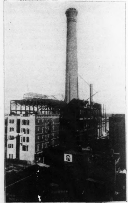
Fig. 5.—The 353-ft. Brick Chimney of the New Power Station of the Metropolitan Traction Co., New York City.
