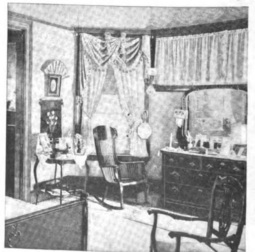
Light at a Bureau is secured in a bedroom of a California home by the expedient of cutting a window through the wall just over the mirror.
