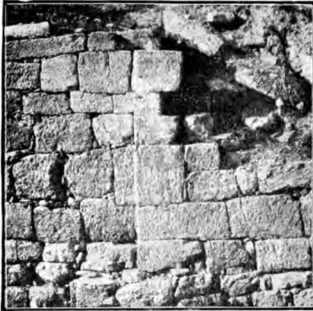
FIG. 9. RETAINING WALL OF VI M
