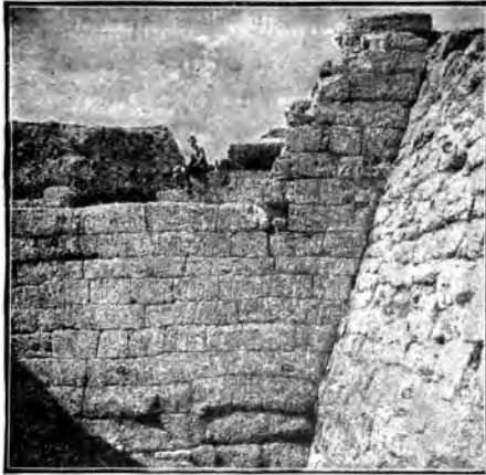
FIG. 10. NORTH WALL OF TOWER VI h
