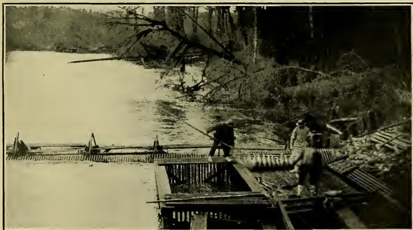
FIG. 2.—CHEHALIS HATCHERY, WASHINGTON FISH AND GAME COMMISSION, SHOWING RACKS TO PREVENT SALMON FROM GOING UPSTREAM AND PEN FOR HOLDING SPAWNING FISH.
