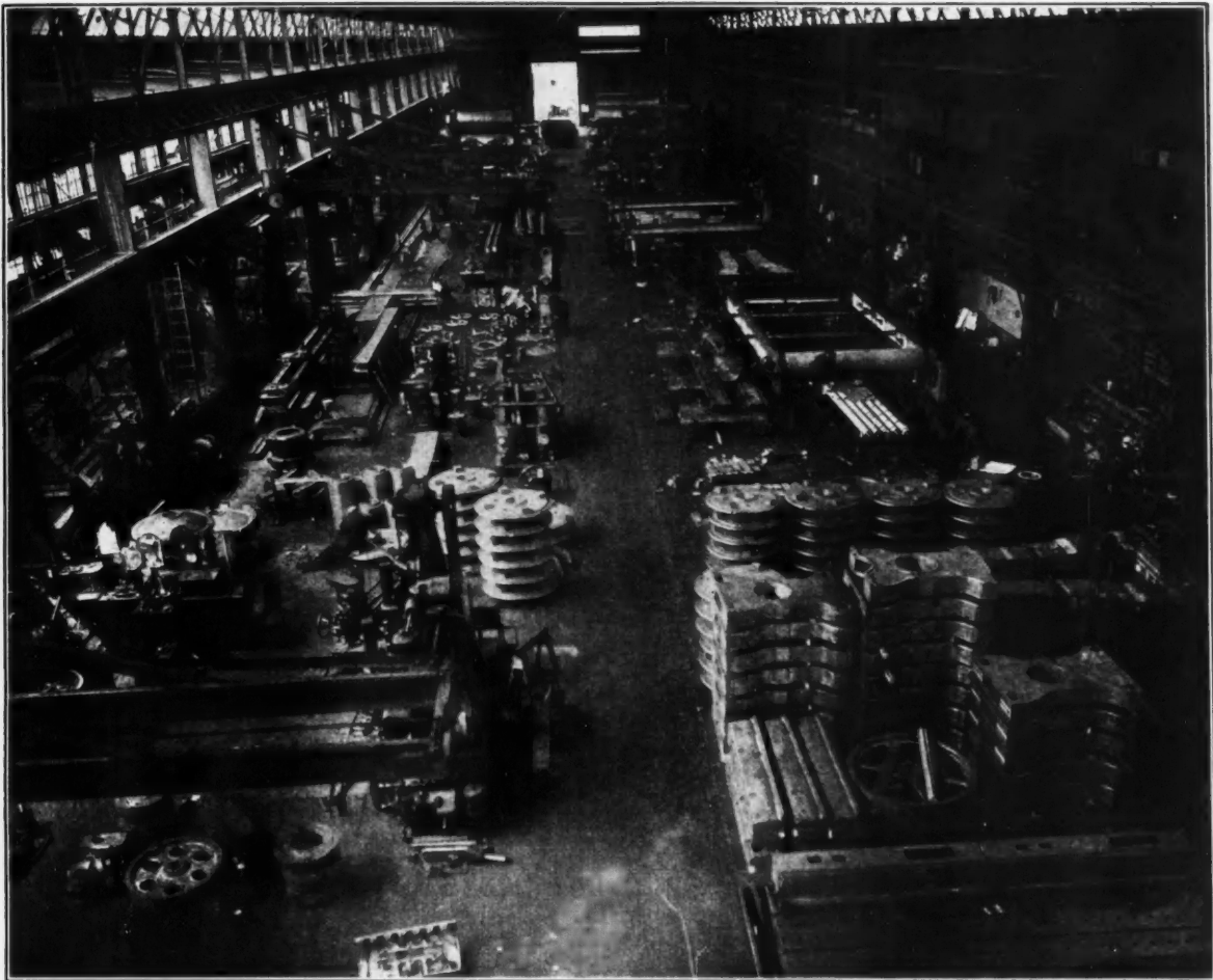
View of Main Erecting Floor
