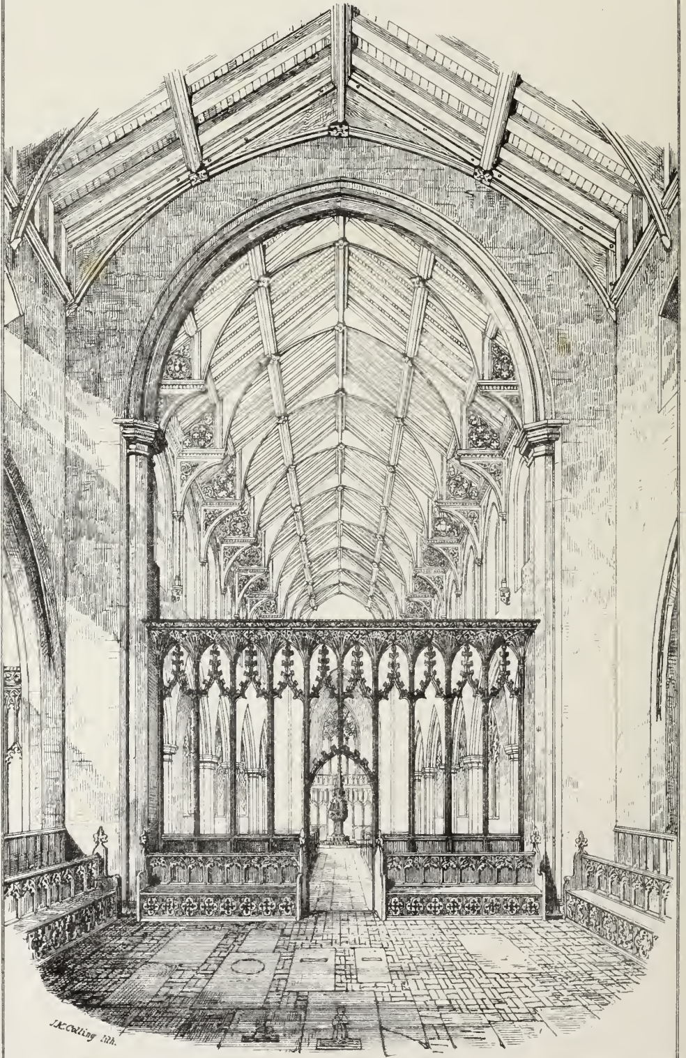
INTERIOR OF WORSTEAD CHURCH, NORFOLK.
