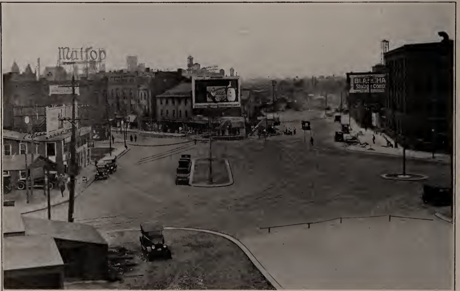
MAIN STREET W AND CALEDONIA AVENUE BRIDGES REMOVED—SHOWING NEW SUBWAY STREET CONSTRUCTION
