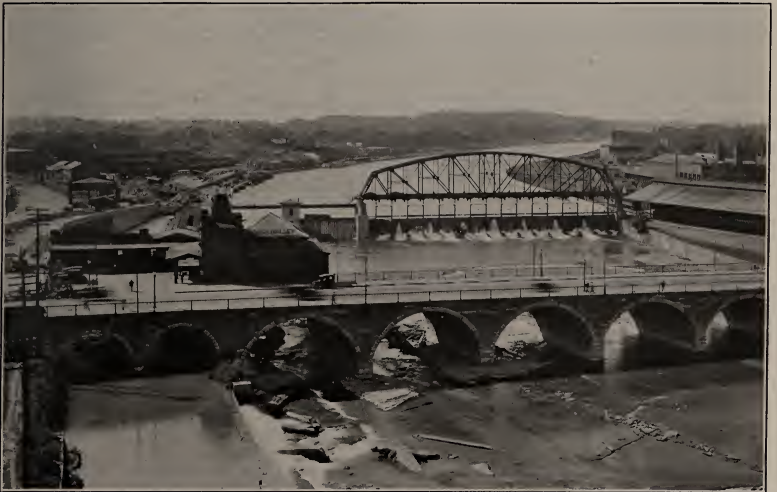
BARGE CANAL—COURT STREET DAM—ROCHESTER HARBOR
