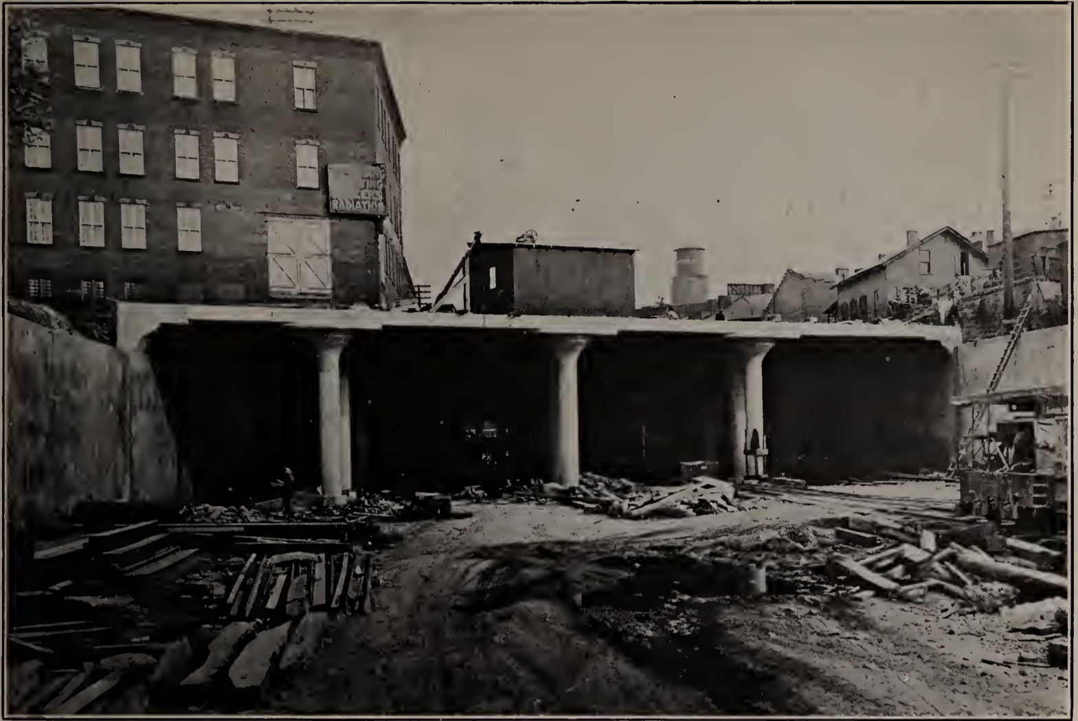
ENTRANCE TO COVERED SECTION OF SUBWAY AT OAK STREET
