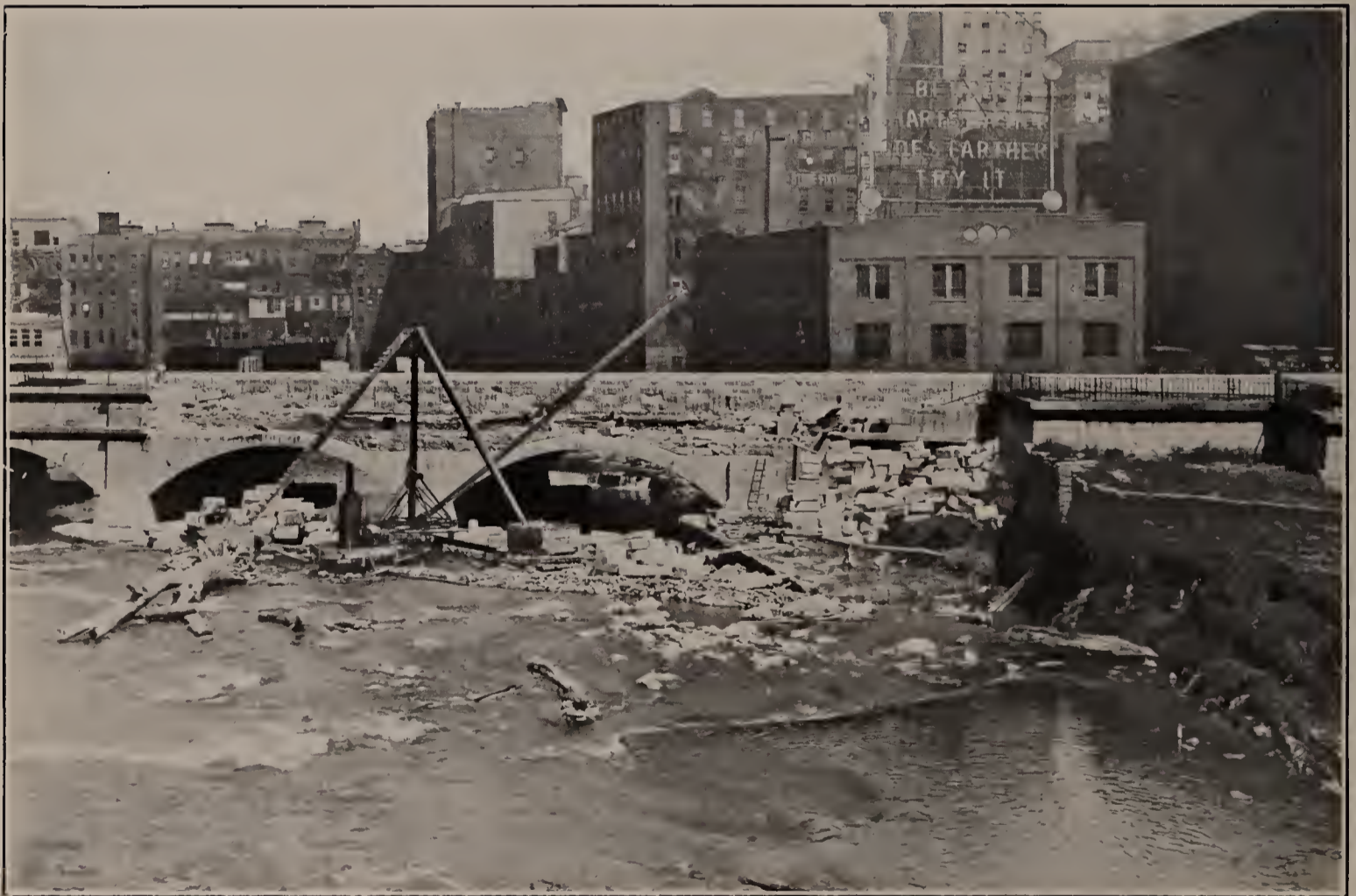
EXTENDING TWO EASTERLY ARCHES OF THE AQUEDUCT ACCOUNT OF SUBWAY CONSTRUCTION
