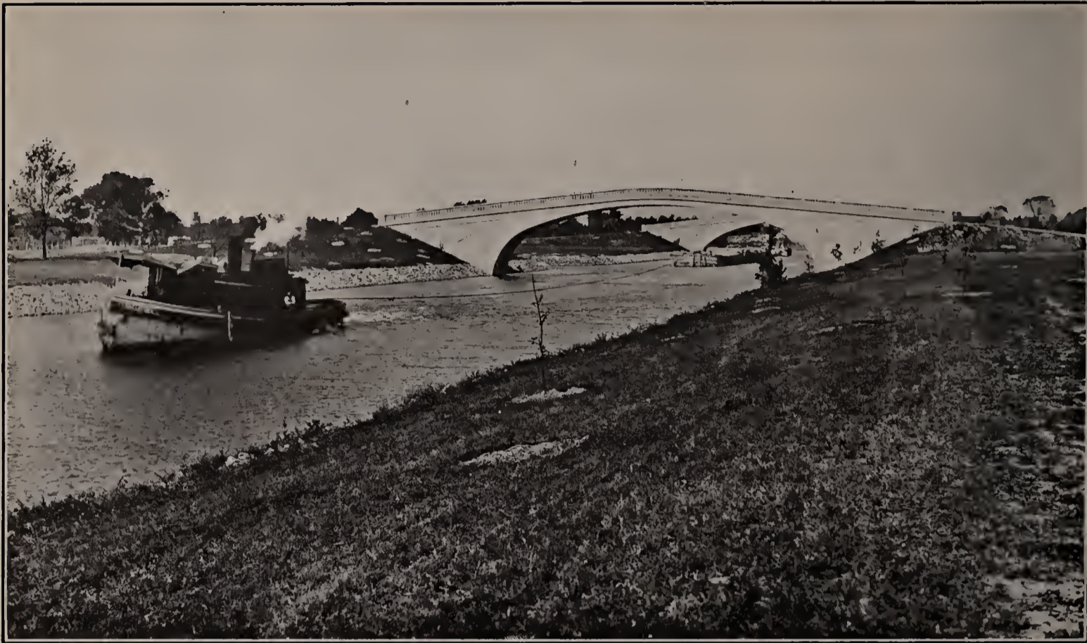
GENESEE VALLEY PARK—NEAR VIEW OF FOOT BRIDGES OVER BARGE CANAL
