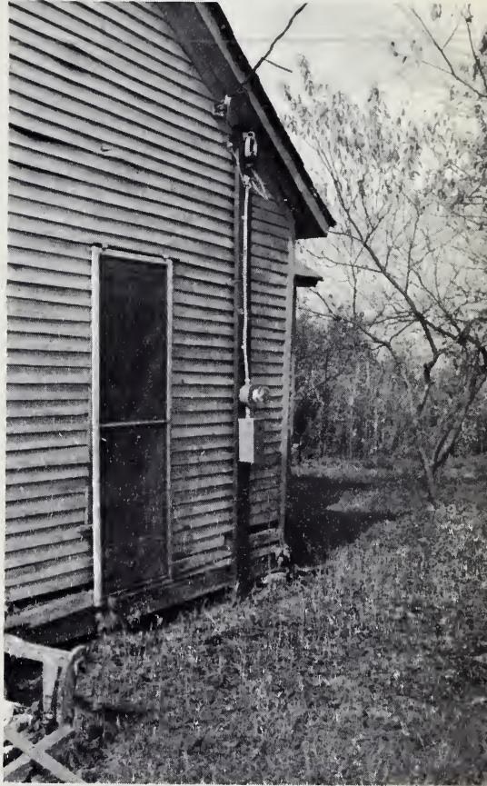
Idle service on a tenant house.
