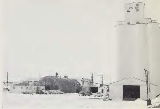
Grain elevator and safflower processing plant are industrial loads.
