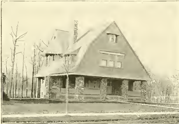
RESIDENCE GEO. W. NIX, ESQ.
