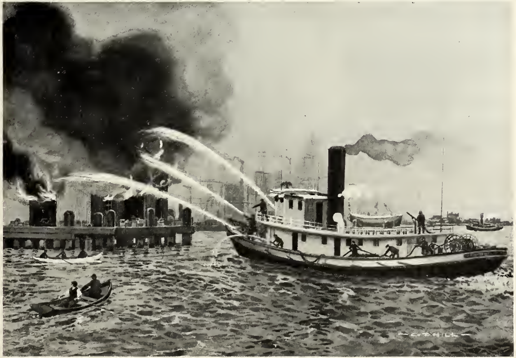
THE FIRE-BOAT, "WM. F. HAVEMEYER," BEGINNING WORK ON A BURNING PIER.
