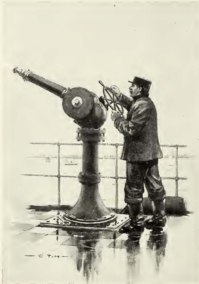
GIANT MONITOR NOZZLE ON THE FIRE-BOAT "NEW YORKER."
