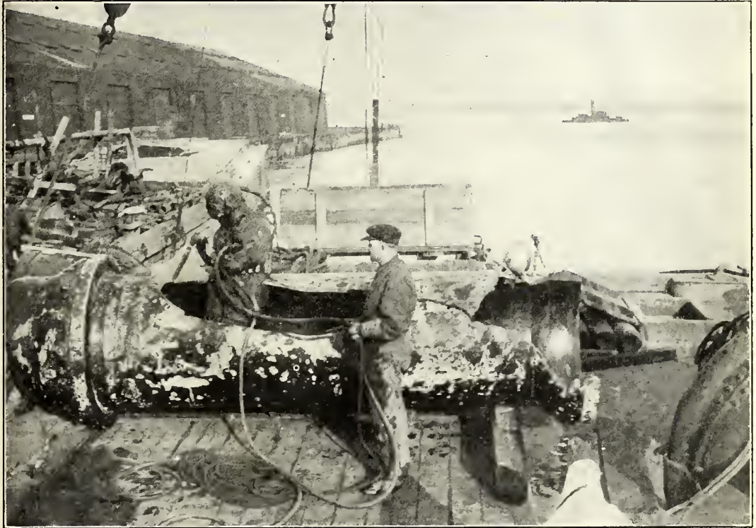
ONE OF THE DIVERS WITH THE CUTTING TORCH IN HIS HAND, SHOWING HOW IT WAS USED UNDER WATER
