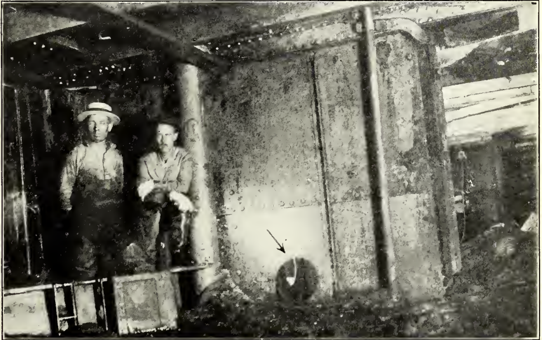
J. W. KIRK AND RALPH E. COLEMAN, INVENTORS OF THE "FLAME THAT WILL BURN UNDER WATER." PHOTOGRAPH TAKEN IN THE "ST. PAUL." THE ARROW POINTS TO THE HOLE MADE BY THE UNDER-WATER TORCH
