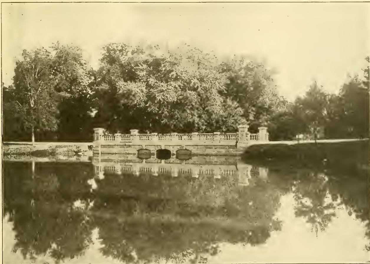
A BRIDGE AT THE NATIONAL SOLDIERS' HOME, WASHINGTON, D. C.
