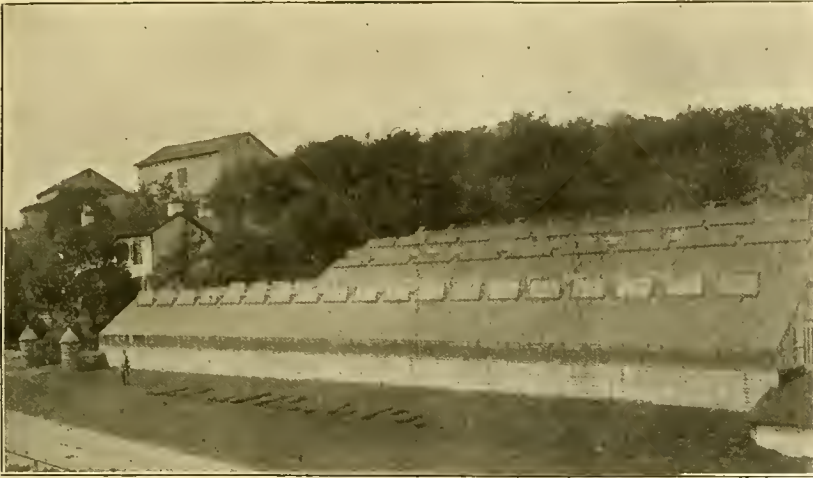
PARTIAL VIEW OF JOHN L. WYLAND'S RANGES, DE HAVEN, PA.
