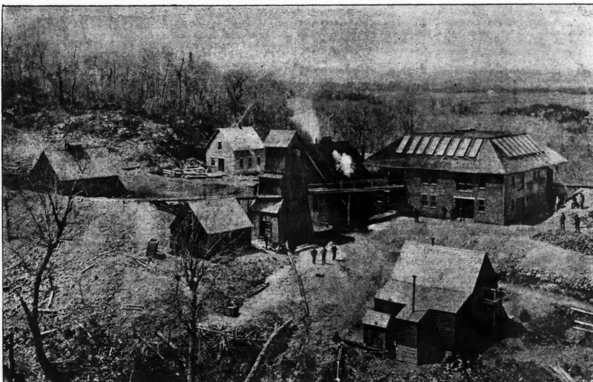
COXHEATH COPPER MINES, NEAR SYDNEY, CAPE BRETON, NOVA SCOTIA.—VIEW AT NO. 2 SHAFT.
