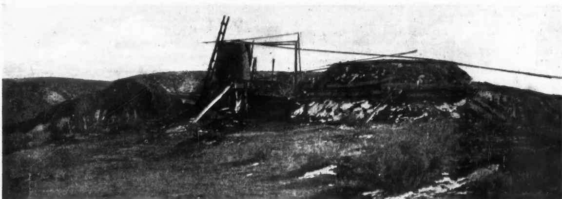
STORAGE TANKS BANKED IN EARTH, CAPACITY, 1,000 BBLs.
