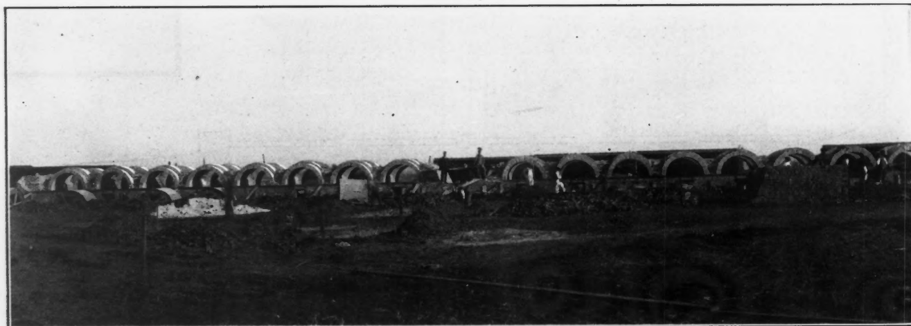
FURNACES IN COURSE OF CONSTRUCTION
