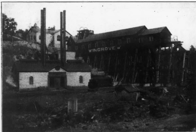
A TYPICAL SOUTHERN WEST VIRGINIA PLANT
